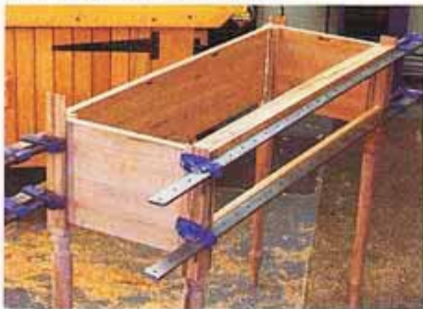
25 Glue and cramp the long rails into the end frames.
